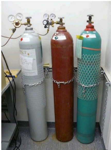
Figure 22: Rules to follow during use. Maintain an exclusion zone around the cylinder. Don't remove valve guards. Use gas regulators. Always restrain cylinders at 1/2 or 1/3+2/3 height. Gas cylinders
